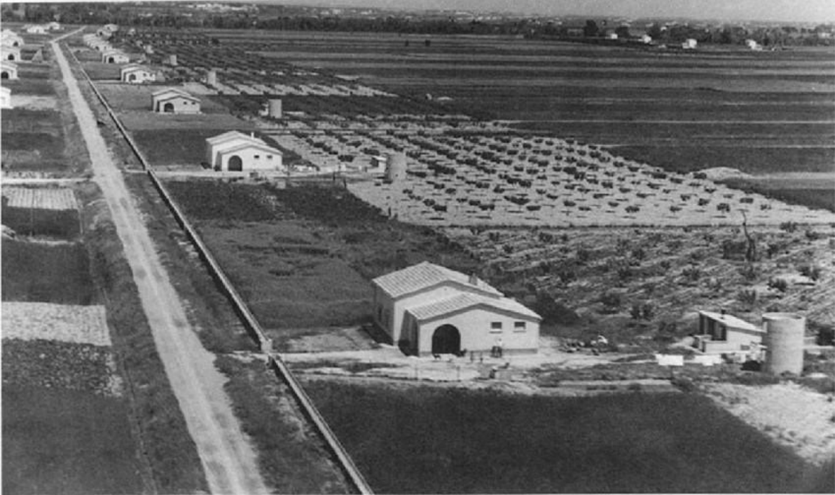
Farming houses of La Martella neighbourhood, Italy, 1951 Source: Rural modernity in post-war Southern Italy: the La Martella village in Matera, Tenzon, 2018
